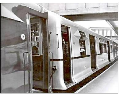
**Above:** A four-car train of Pre-1938 Tube Stock arrives at Acton Town in the early-1950s. The Piccadilly Line's trains were never converted to passenger door control but because of line transfers over the years, some cars had PDC but isolated. The leading 1926/27 motor car is one such car to have the buttons fitted.
